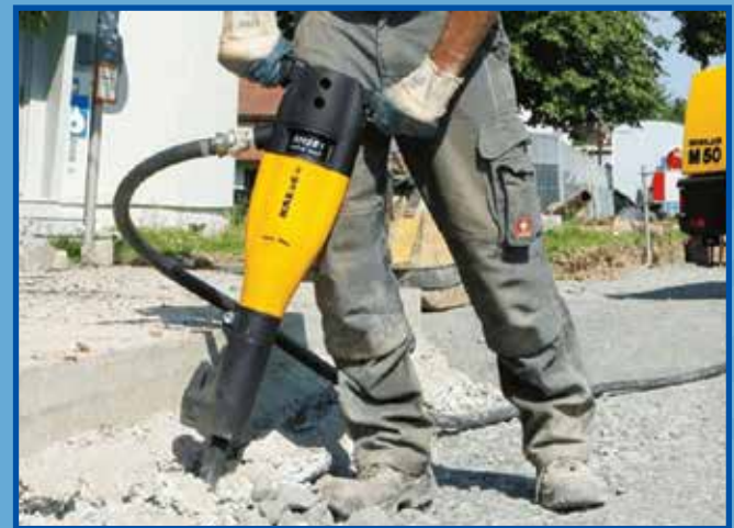
Air Compressor with Breaker
